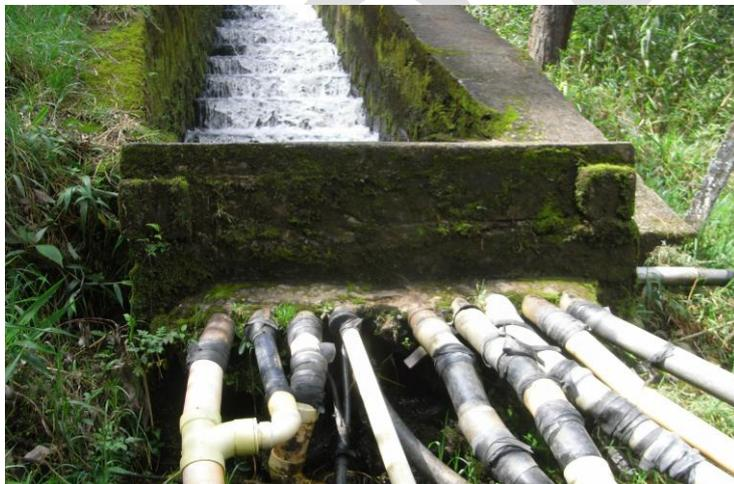
Figure 1. Alternative infrastructure built by inhabitants of Bello Oriente to capture raw water that overflows a tank of the company
